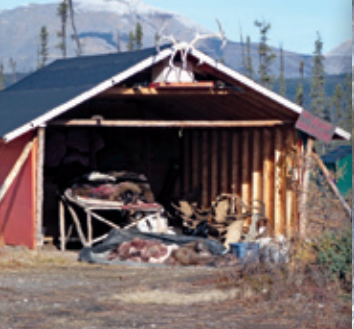
Filling the shed
